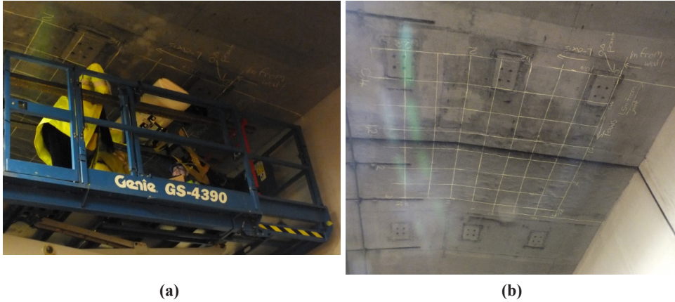
Figure 4. (a) GPR Installation on the Site, (b) Case Study Survey Area
