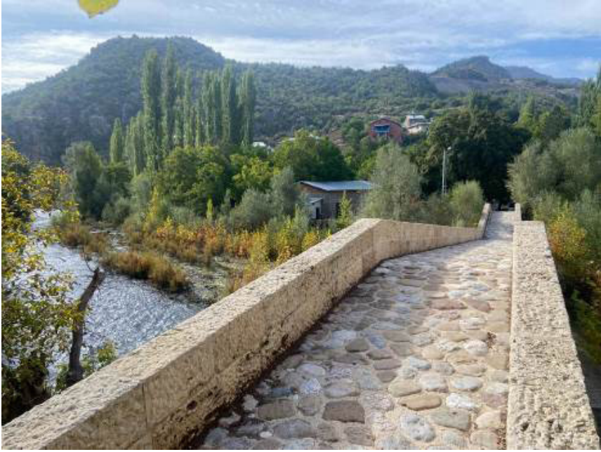
Photograph 8: Sazak Taşkent Üçköprü Bridge
