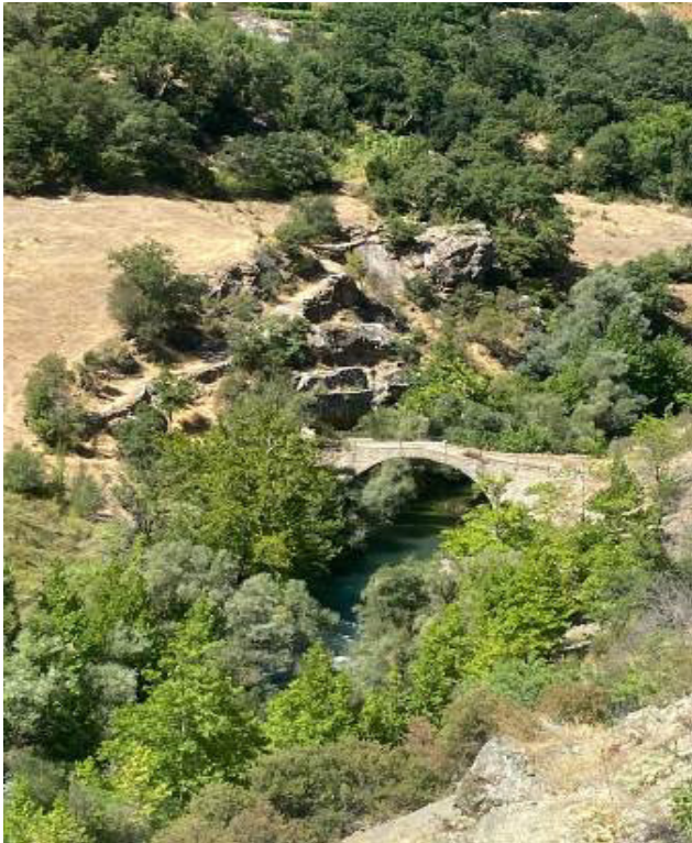
Photograph 9: Korucu (Sucular) Bridge
