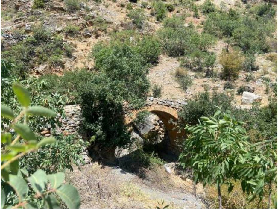
Photograph 6: Korucu (Sucular) Bridge
