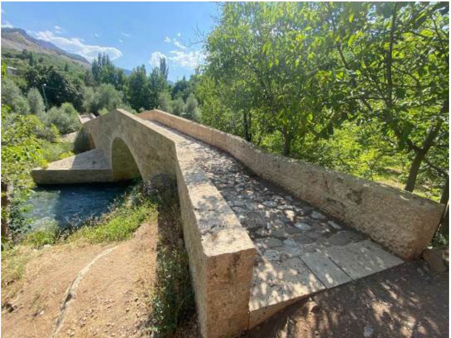
Photograph 7: Sazak Taşkent Üçköprü Bridge
